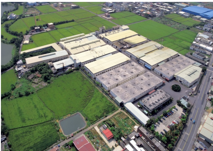
Sheng Hung facilities in Taoyuan, Taiwan.
