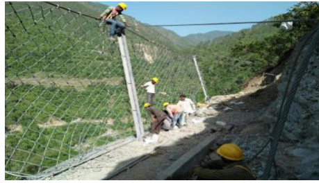
Rockfall protection works using Netting and Rockfall barrier
