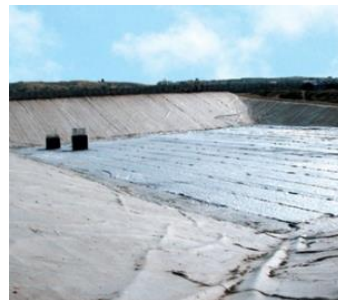
Geosynthetics in Hazardous waste Landfill
