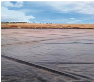
Geosynthetics in Canal Lining
