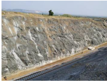
Rockfall protection works using Netting and Rockfall barrier
