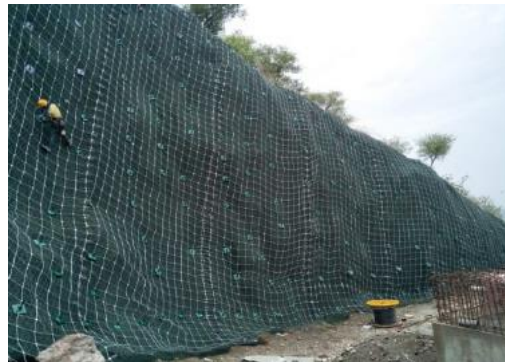
Erosion control using Geosynthetics- Erosion control mats
