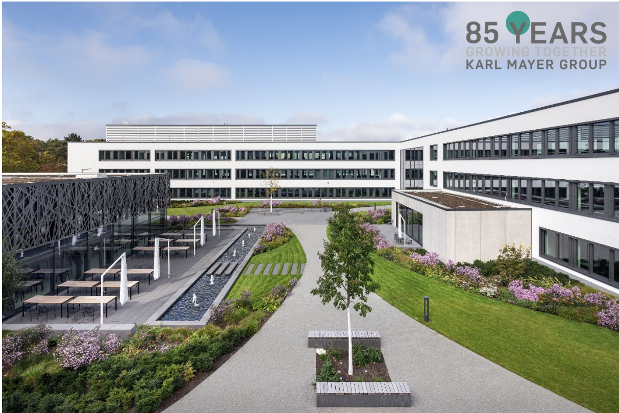
Fig.: The new headquarters of the KARL MAYER Group in Obertshausen
